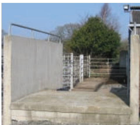
It is a good idea to build a plinth to assist in loading cattle
