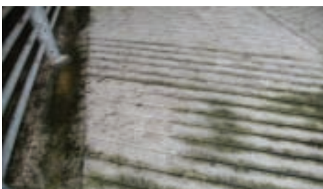
Grooved concrete is less slippery
